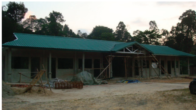
Timimbang Rainforest Lodge (TRL) under construction
