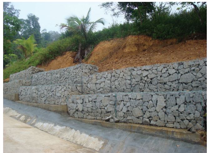
Reinforcing of road using gabiion embankment.
